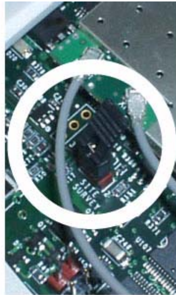
B. Site Survey Jumper Installed
