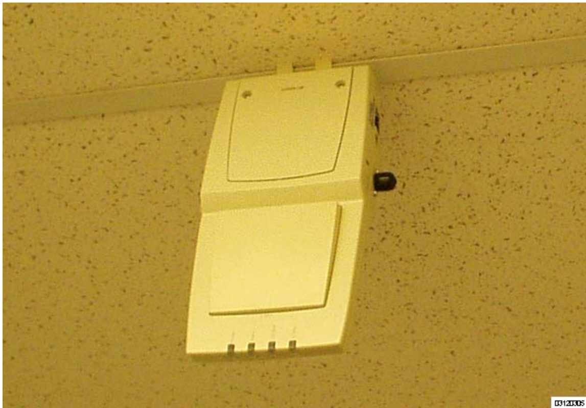
Figure - Clipping the Airespace AP and Ceiling-Mount Clips to a Hanging-Ceiling Rail
