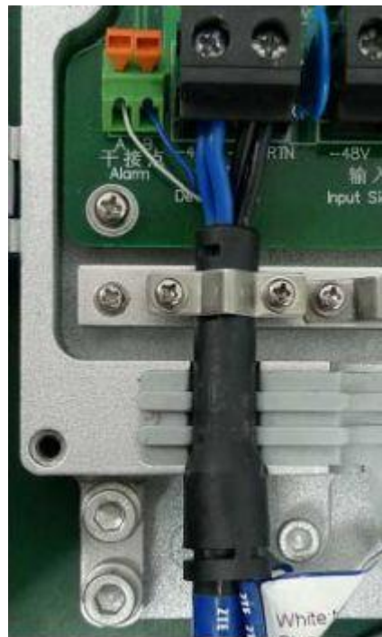
Figure 2-37 PIMDC Connection (to LMKT RL1F22)
