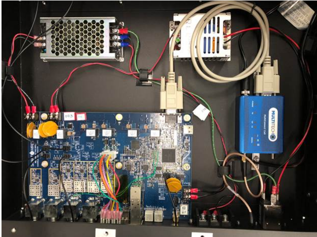
PLC enclosure top view with cover removed, high-level assembly.
