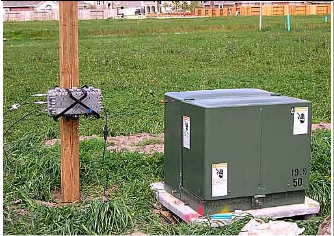
Unit and Coupler Installation with Transformer Door Closed
