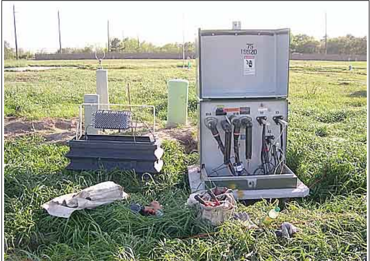
Initial Installation of Coupler
