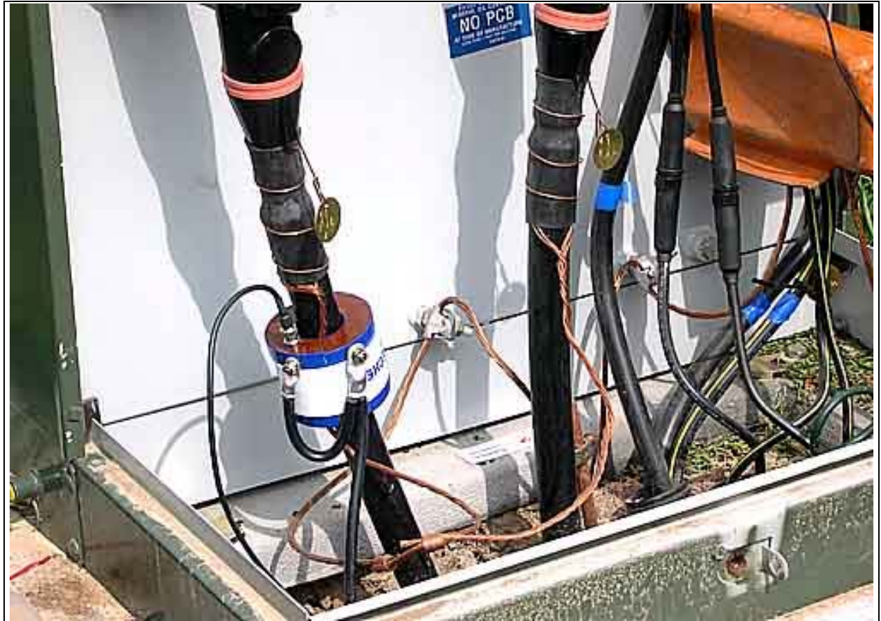
Coupler Installation Closeup
