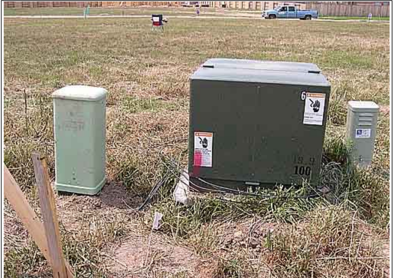
Underground Site with Cover Installed
