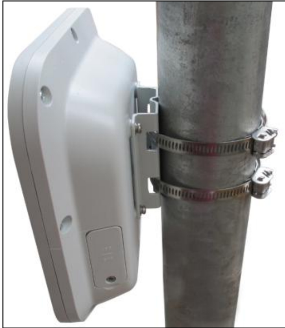
Figure 3-6 The installation is complete
