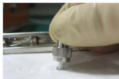
Figure 5-96 Cleaning optical fibers with special cleaning tissues
