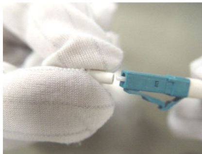
Figure 5-99 Installing a protective cap on a fiber
