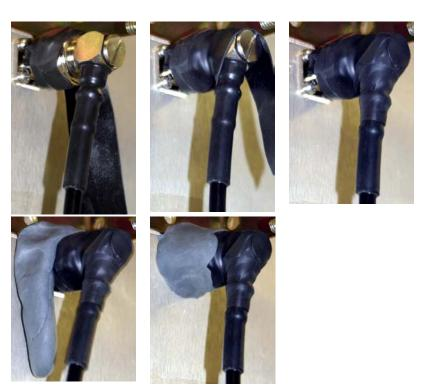
**Figure 15 Waterproofing Outdoors Connections**
