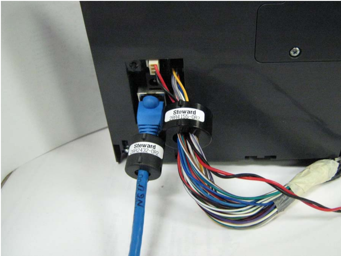
Figure 4-16: Installation of Ferrite Cores
