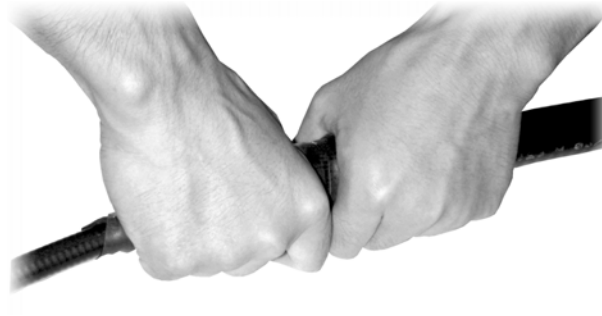
Fig. 10.6-3 Wrapping the Waterproof Adhesive Tapes (3)
