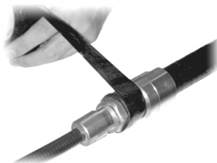
Fig. 10.6-1 Wrapping the Waterproof Adhesive Tapes (1)
