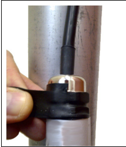
Figure 2-25: Applying sealant tape to an external connection
