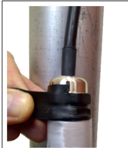
Figure 2-42: Applying sealant tape to an external connection
