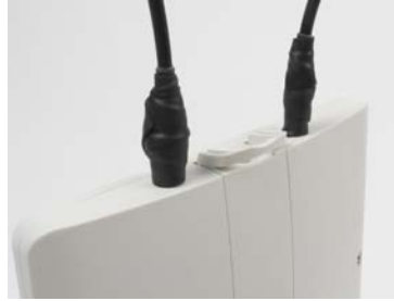
Sealing tape applied
