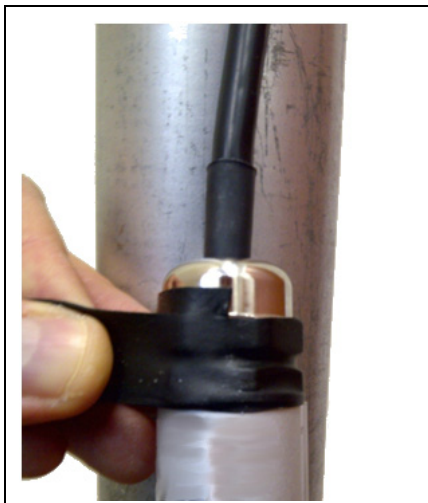
Figure 2-40: Applying sealant tape to an external connection
