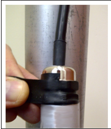
Figure 2-25: Applying sealant tape to an external connection
