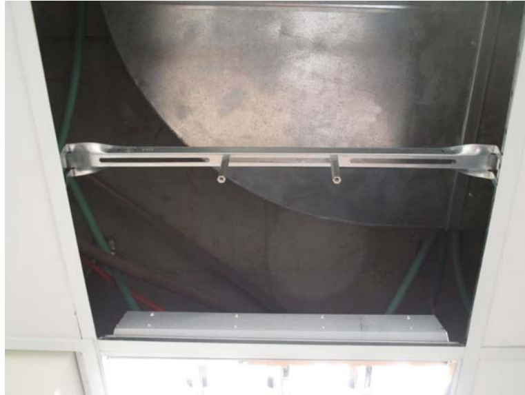
Figure 14: Mounting Clip with Screws and Spacers
