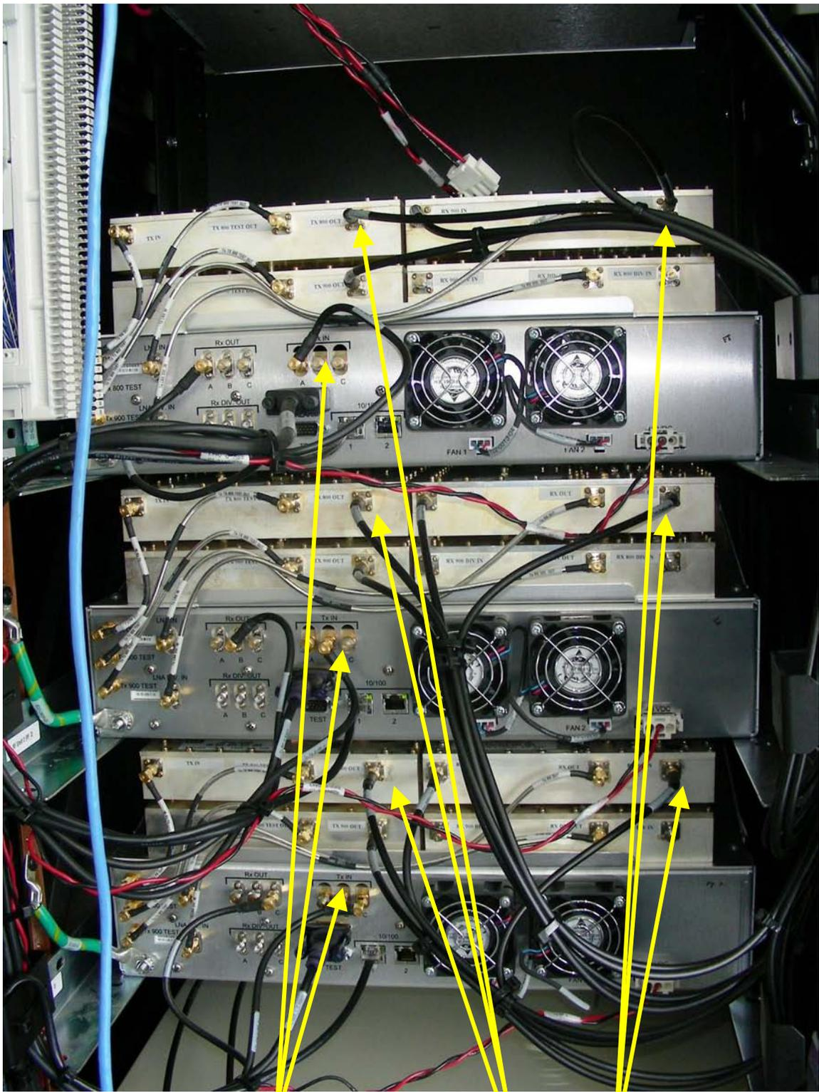
Transmit signal in from Radio in RBS      800 MHz      900 MHz
