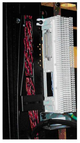
Figure 25 Punch Block Location within the MC-Series Rack
