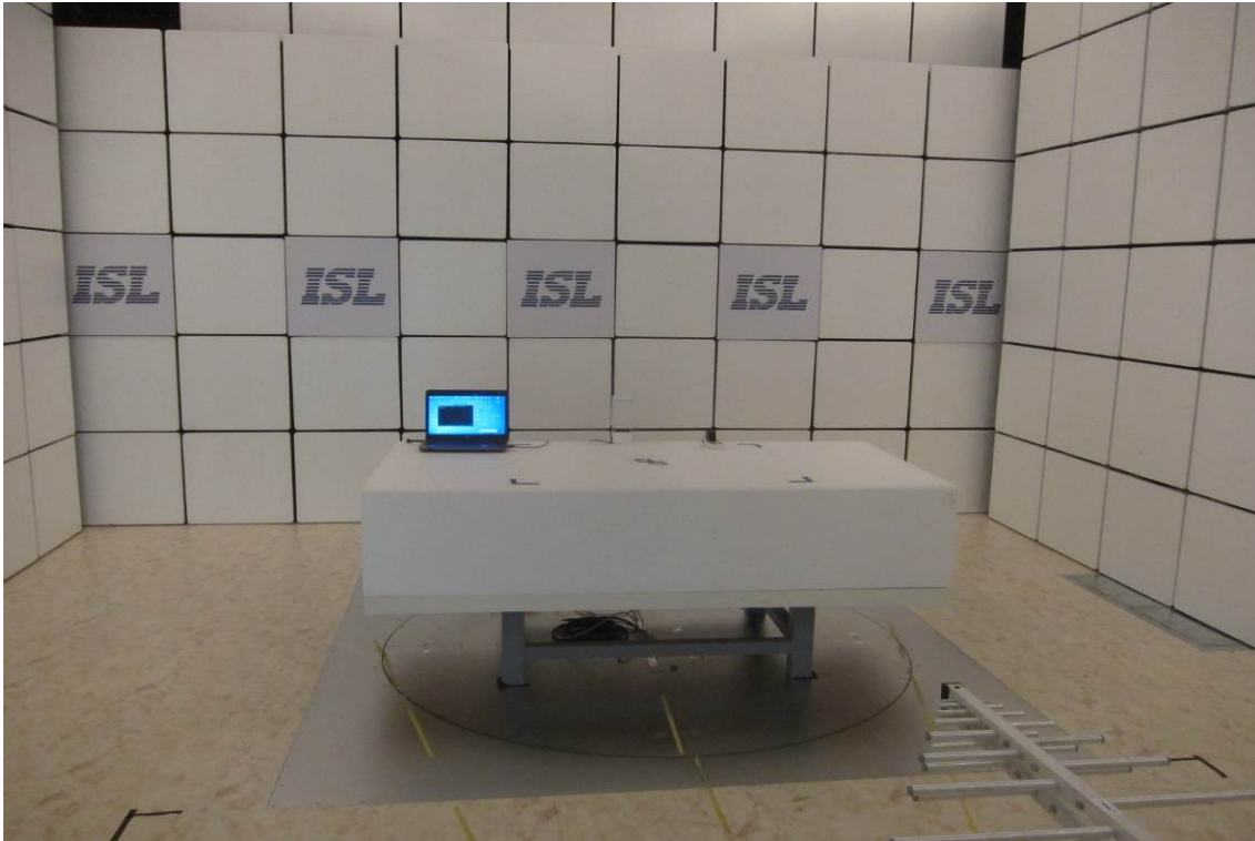
Radiated Emission Set up Photo (under 1GHz)
