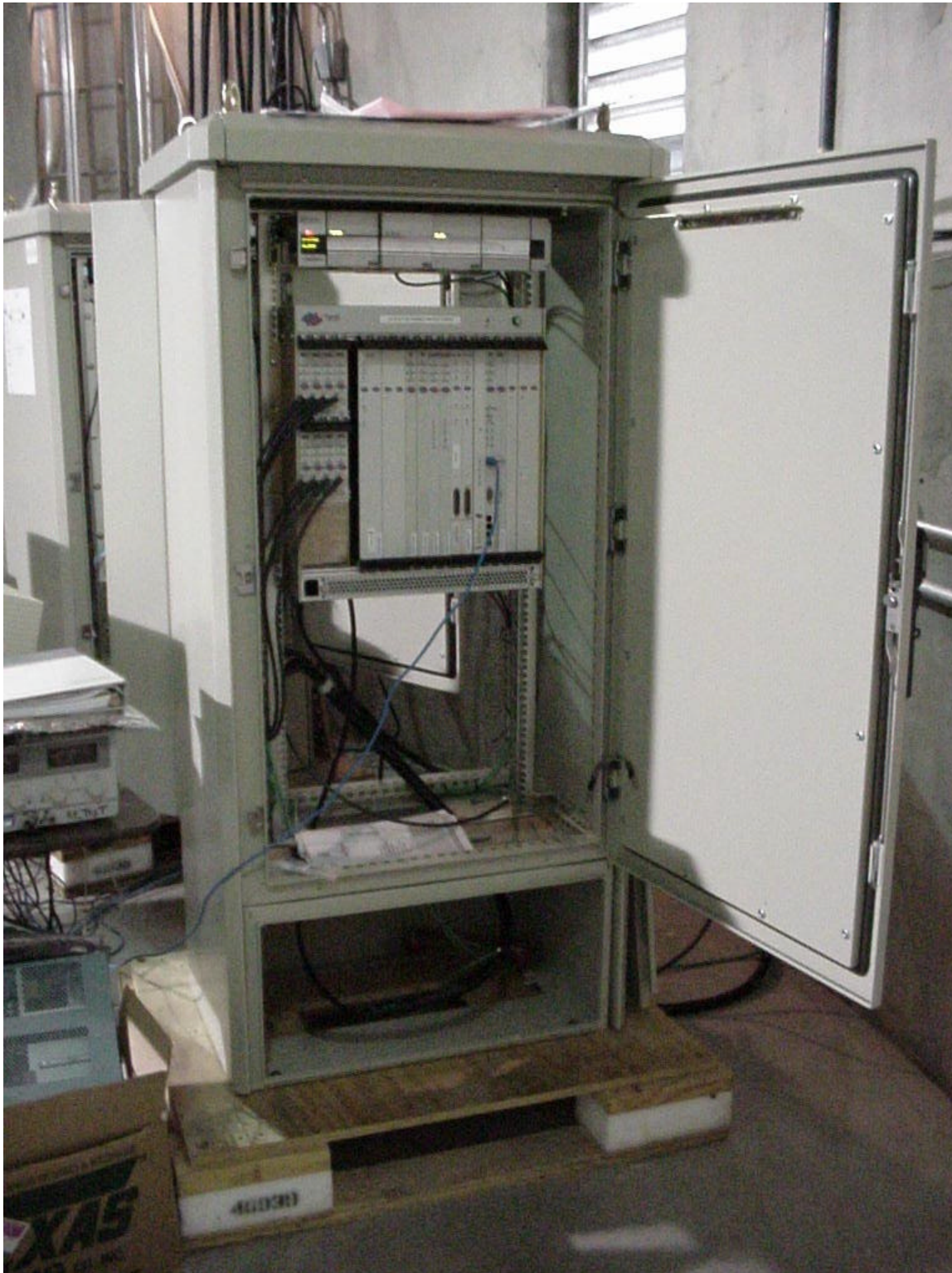
Figure G7: TTA Digital Chassis (Front)
