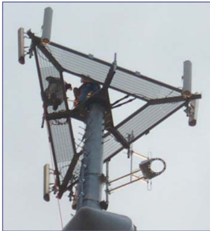
Figure 40: Secured Omni Antenna Mount
