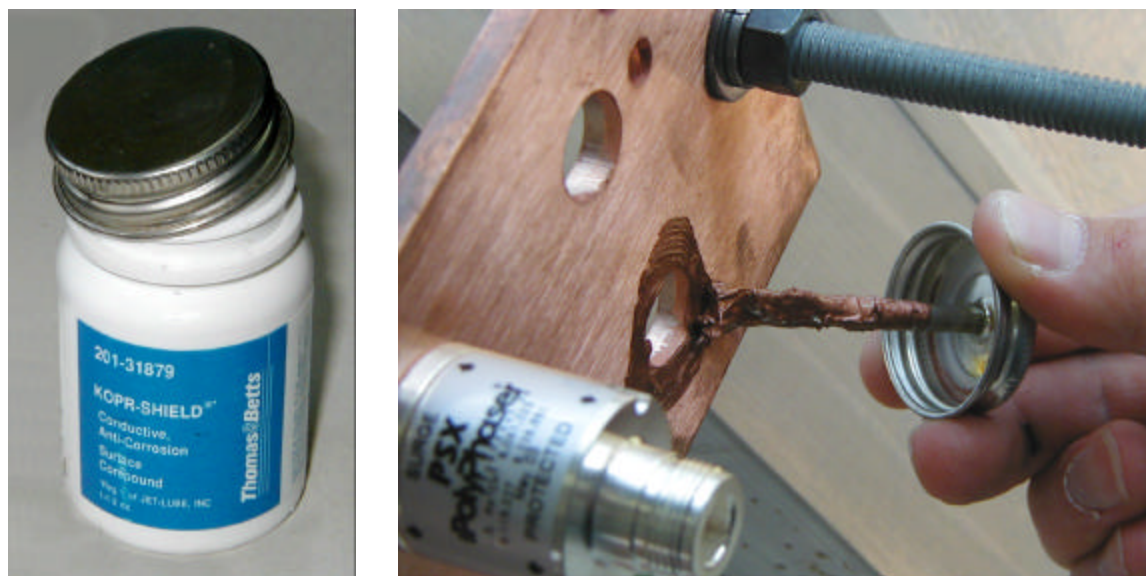
Figure 14: Applying anti-oxidant joint compound
