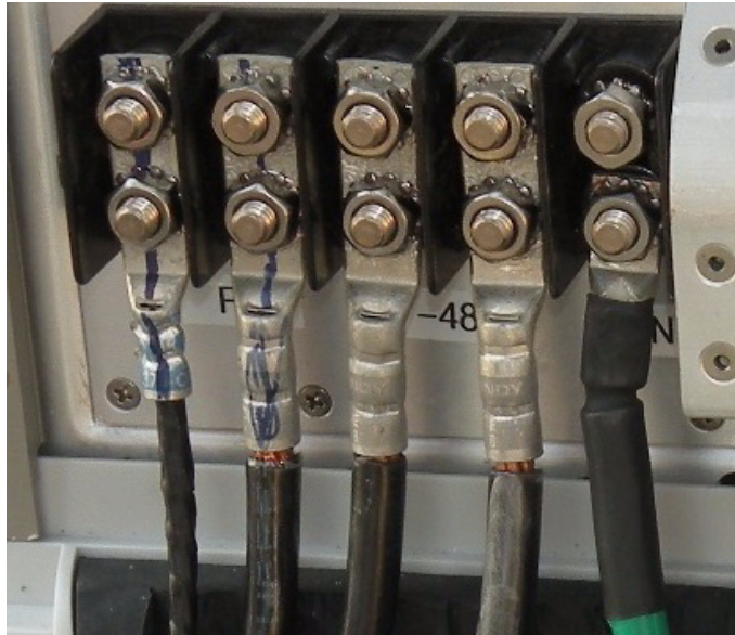
Figure 6-22 Power Cable Leads Installed
