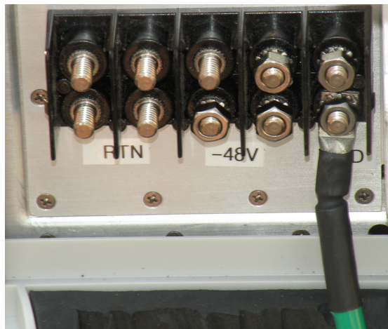
Figure 6-21 Ground Cable Installed
