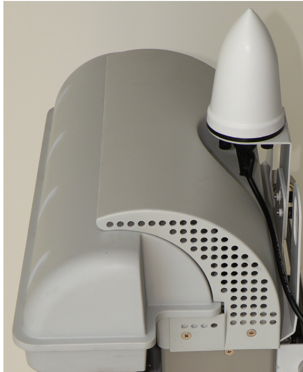
Figure 6-7 GPS Antenna Cable Installed
