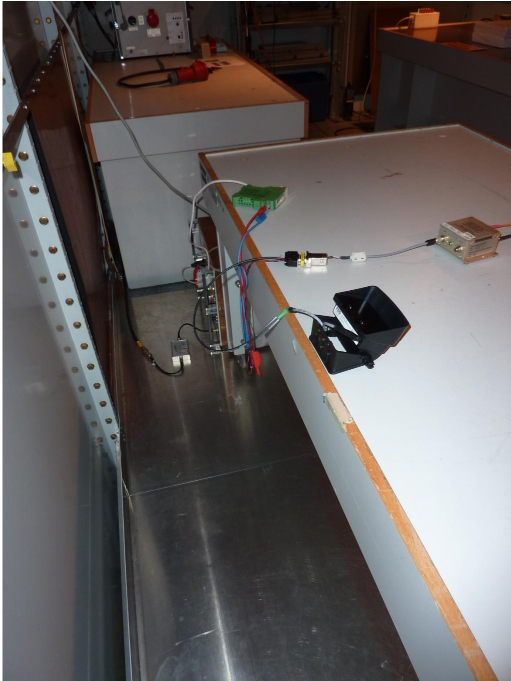
160532_111.jpg: MWD BPC-HU (DC supplied), test setup shielded room
