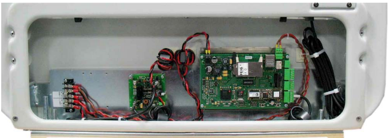
Fig. 9: Tying the cables
