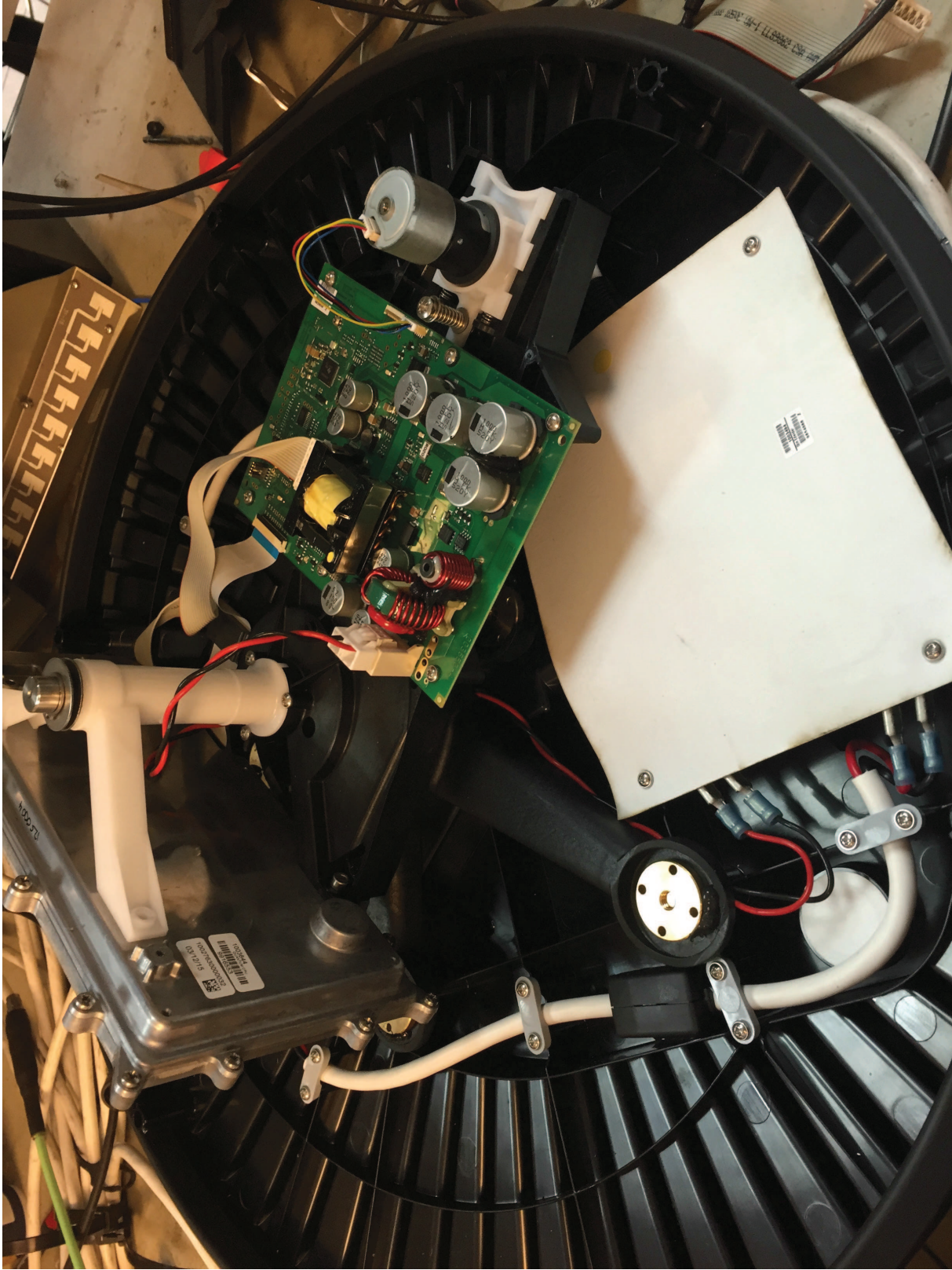
Figure 1 – Radar – dome cover removed
