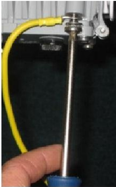
Figure 25 – attaching ground cable to AirSynergy
