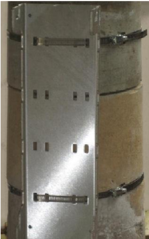
Figure 14 – mounting plate installed on large diameter pole
