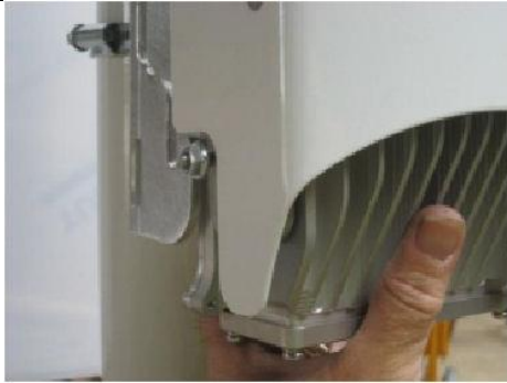
Figure 23 - lift the unit until the bottom studs fit into the bottom slots
