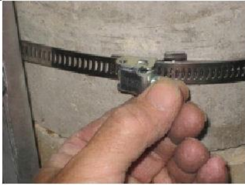
Figure 12 – press down locking mechanism
