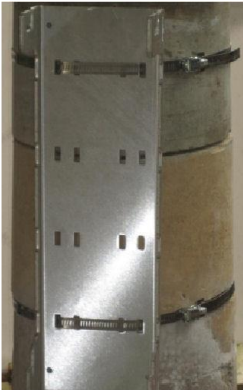
Figure 14 – mounting plate installed on large diameter pole
