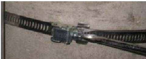
Figure 13 – tighten clamp bands
