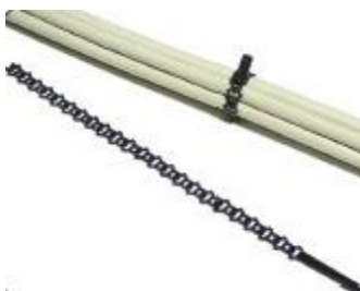
Figure 42 – Secure fiber-optic cable, cut excess tie
