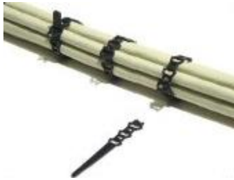
Figure 51 – Secure fiber-optic cable, re-use excess tie
