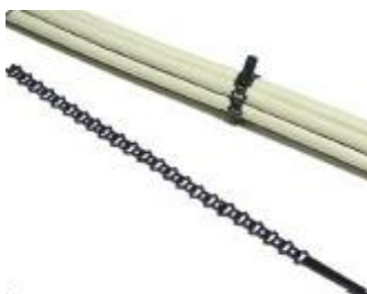
Figure 49 – Secure fiber-optic cable, cut excess tie
