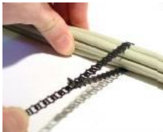
Figure 48 – Secure fiber-optic cable, pull tie
