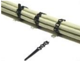
Figure 52 – Secure fiber-optic cable, re-use excess tie
