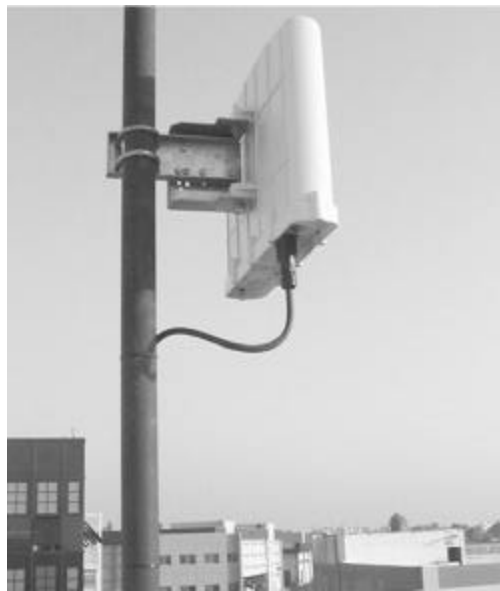
Figure 4-1: Typical BSR Installation
