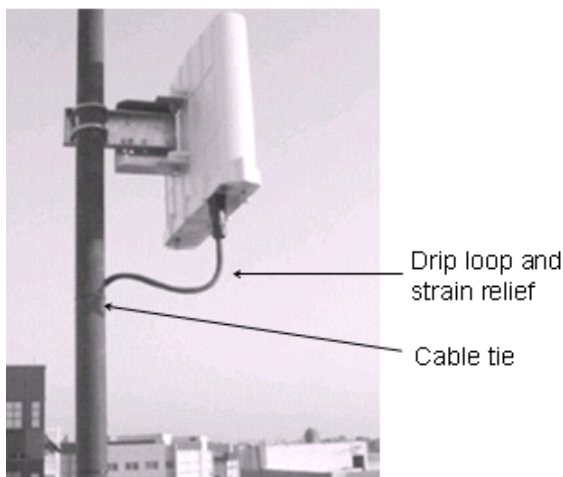
Figure 29 - strain relief
