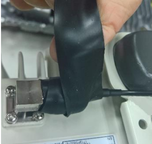
Figure 9: Weather-proof the GPS Connection
