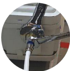
Figure 13: Use 2 Wrenches to Loosen
