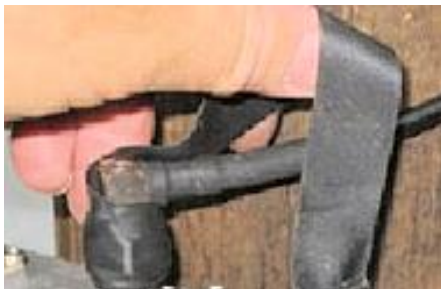
Figure 11: Weather-proof the Connection
