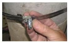
4. Wrap the band to properly fit on the pole. Press down locking mechanism with band excess fed through the mechanism.
