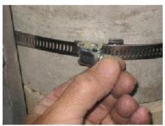
6. Align and position each of the 4 pole clamps. Tighten the clamp bands with large flat screwdriver in place.
