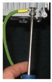
Connect the ground cable to the protection ground bar using suitable crimp lugs.
