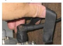
2. Weather-proofing of the RF N type connections is recommended. This is done with a layer of self-amalgamating tape followed by an over layer of PVC tape.
