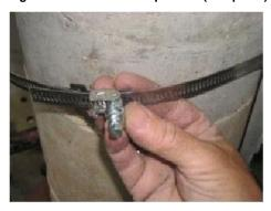
5. Wrap the band to properly fit on the pole. Press down locking mechanism with band excess fed through the mechanism.
