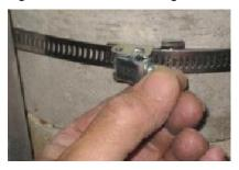
5. Align and position each of the 2 clamps. Tighten the clamp bands with large flat screwdriver in place.
