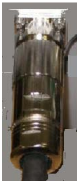
Figure 27: attaching power cable to AirHarmony
