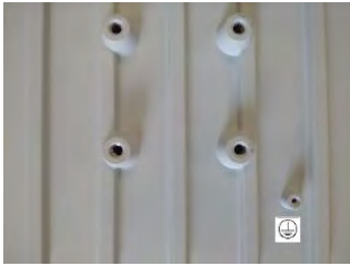
Figure 3-5: Enclosure Ground Connection
