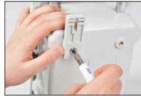
Using a T30 torx screwdriver, turn the torx screw clockwise to tighten.
