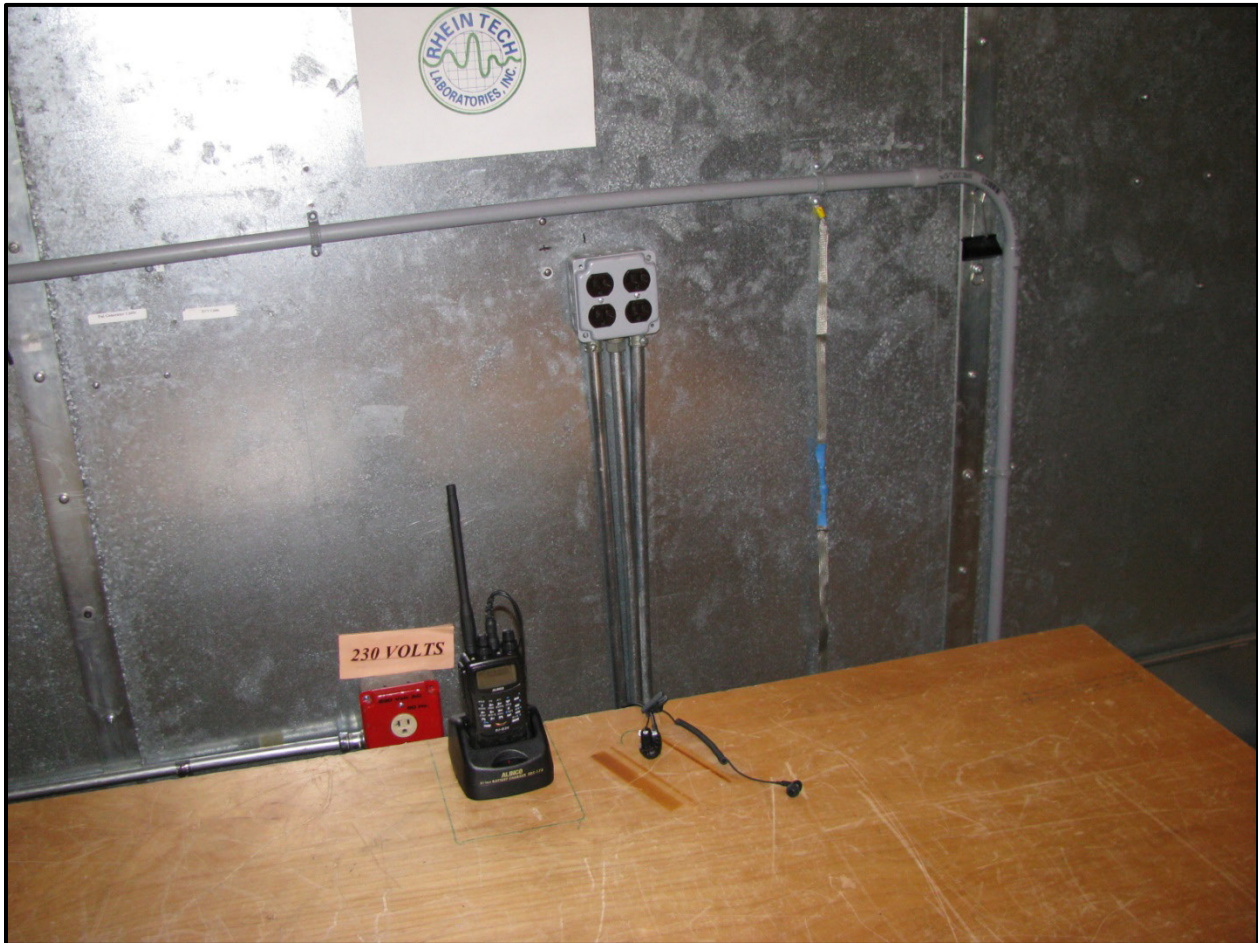
Photograph 4: Conducted AC Emissions Test Configuration (Front View)
