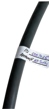
Figure 1.7 – Service End Labeling
