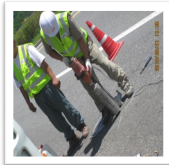
Coring Sensor Hole
