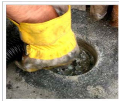
Clearing Sensor Hole
