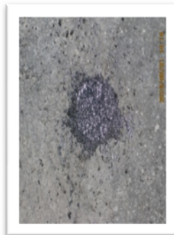
Filling Hole With Epoxy
