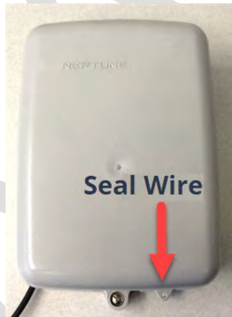
Figure 24 – Installing the Seal Wire
