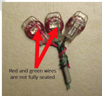
Figure 40 – Improper Connections
