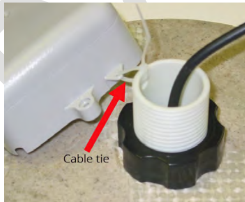
Figure 44 – Attaching the R900 cellular endpoint to the Antenna Shaft
