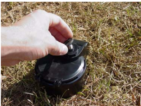
Figure 15 Placing Washer on MIU
