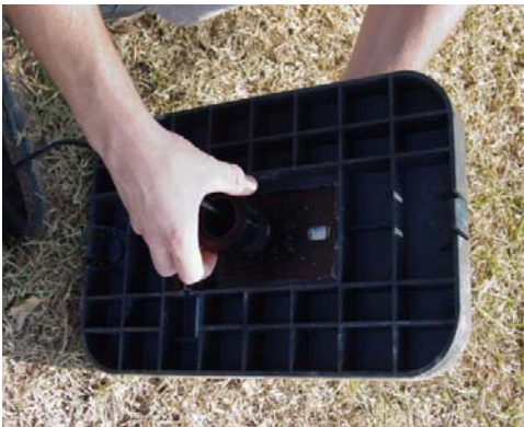
Figure 14 Feeding Antenna Cable
