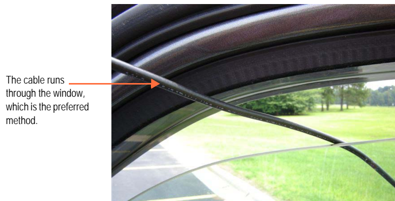
Figure 3.19 Antenna Cable Through Window
