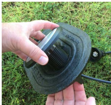
Figure 28 – Inserting the Antenna into the Pit Lid
