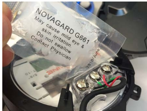
Figure 8 – Application of the Sealant
