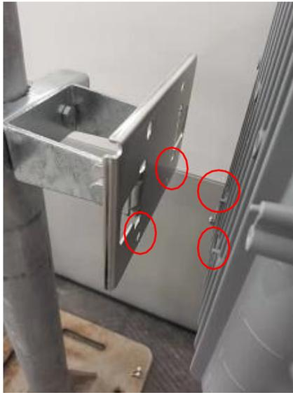
**Align the positioning hole**
