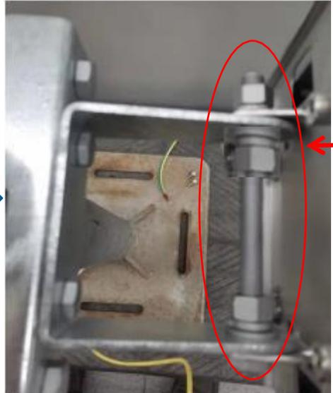
Note the sequence of screw and washer (From M12 Screw pack)
