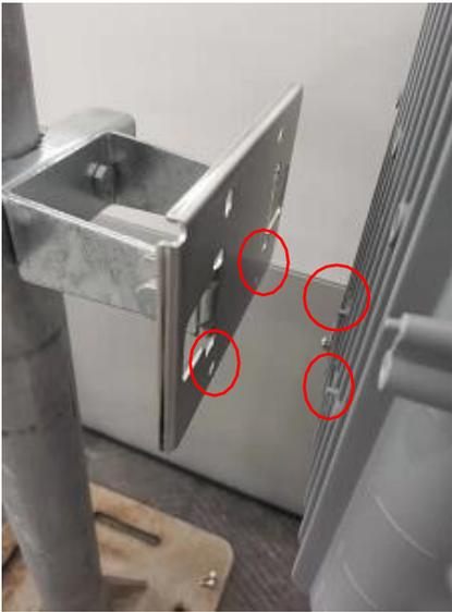
**Align the positioning hole**
