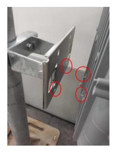
Align the positioning hole
