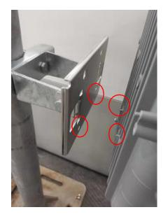
Align the positioning hole
